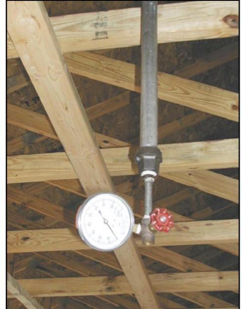
Sprinkler hydrostatic tests are measured at the lowest point of the system or portion of work.
