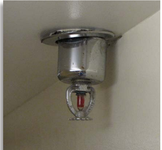
This standard spray pendent sprinkler should be located at least 4 in. (102 mm) from the wall.
